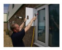
Remove masking tape whilst Protectapeel is still wet.
